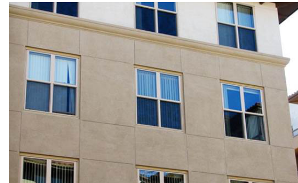
Figure 5.3. Example Expansion Joint Alignment
