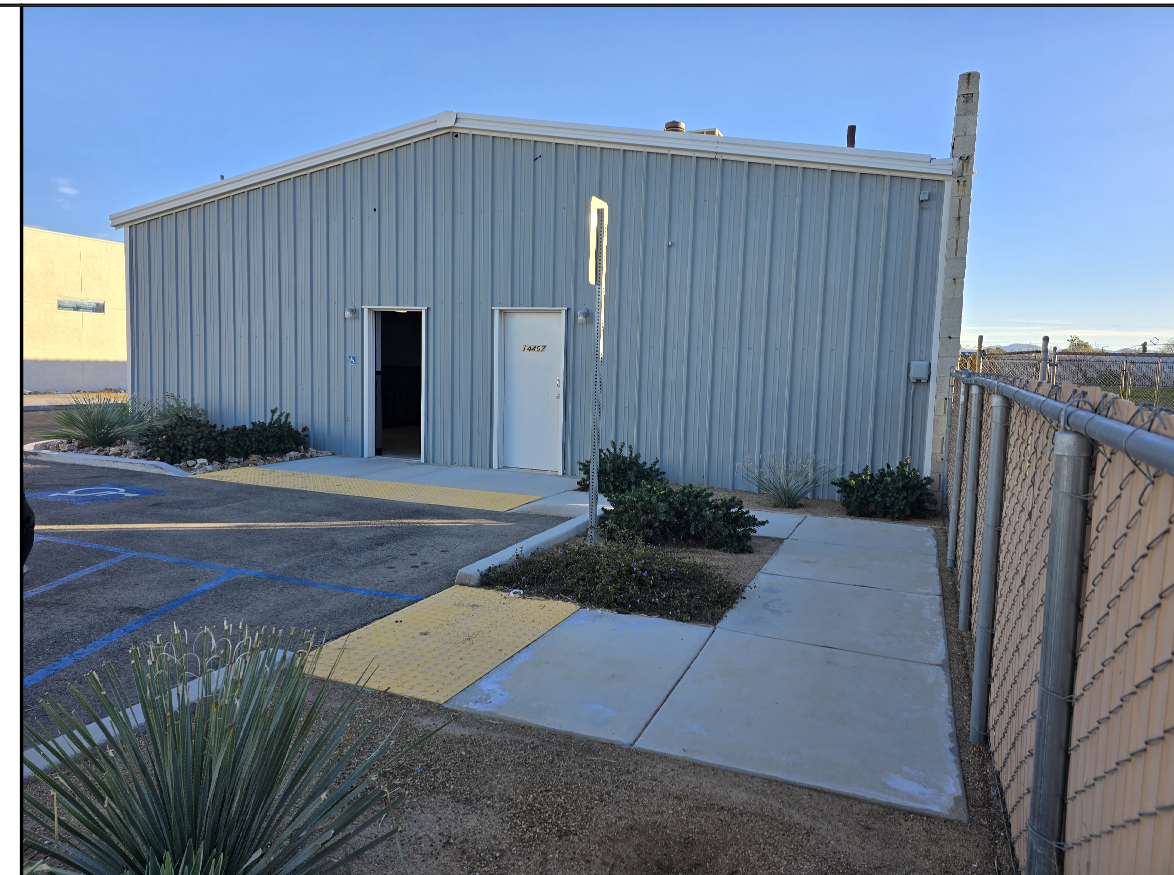
3 View of Exterior - North & Parking Area
