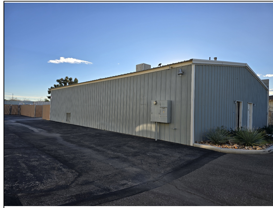
1 View of Exteriors - East & North
